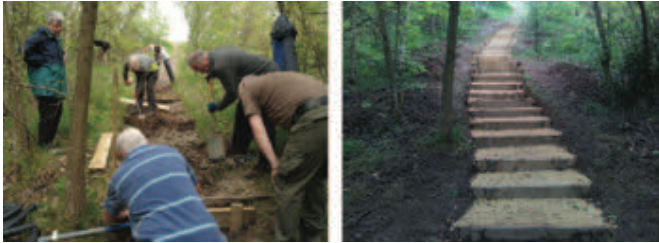
Stepping up to the challenge - Volunteers installing the steps at Ledston Luck and the final product!
